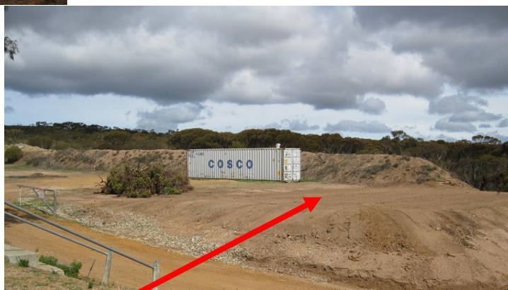
Pad for new 100m range
