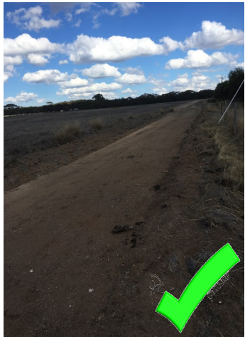
Diagram 4.1; 3 metre wide Bare Earth Fire Break.
