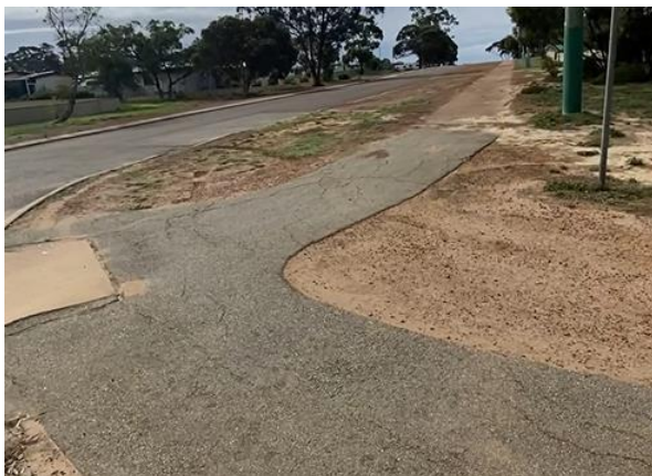
Figure 4-29: Daw Street from Carlisle Street
