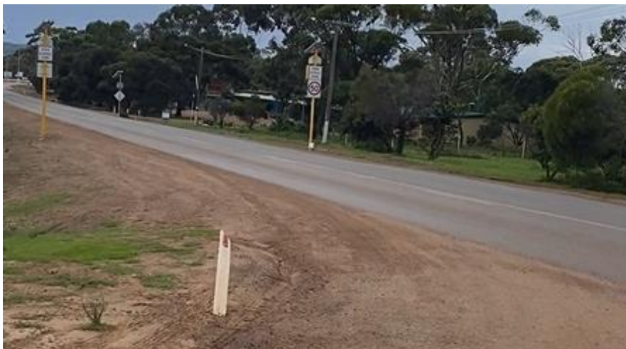
Figure 4-32: Jamieson Street from Elston Street
