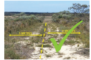
Diagram 7.1; 3m mulched firebreaks
