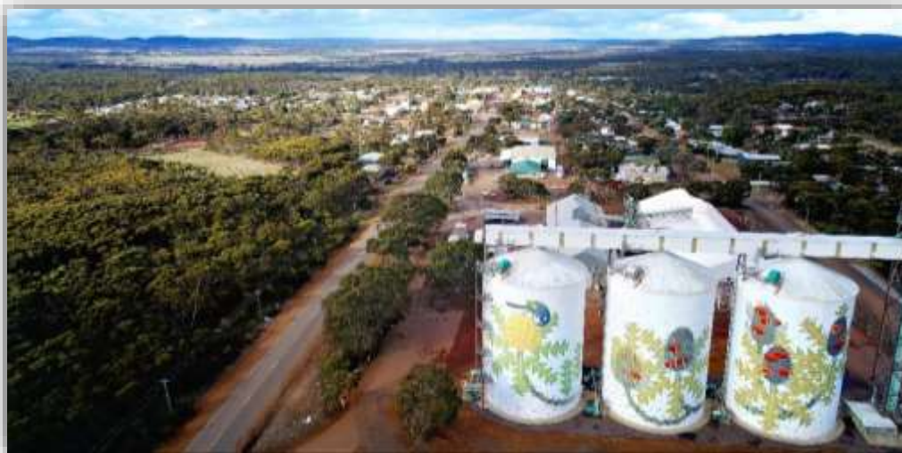
RAVENSTHORPE TOWNSITE - SILOS
