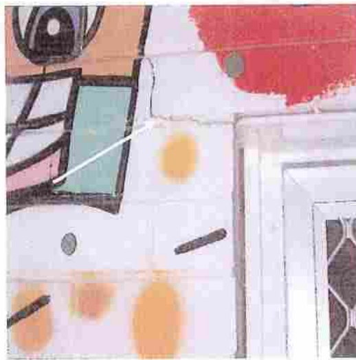
Cracks in External Hardi-Plank Wall Lining
