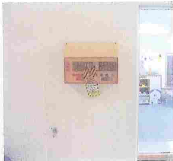
Electrical Sub-Board Tagged Out
