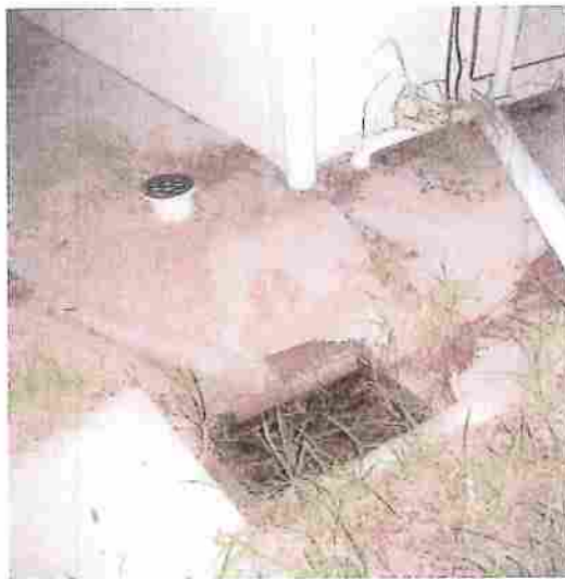
Stormwater Pipe Fitting Leaking
