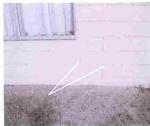
Cracks in External Hardi-Plank Wall Lining
