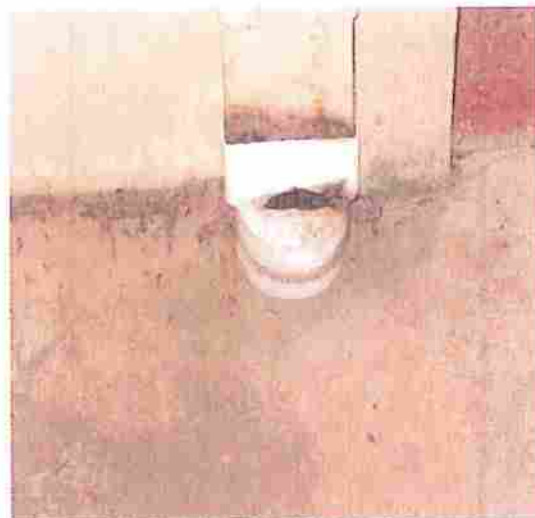
Stormwater Pipe Fitting Leaking
