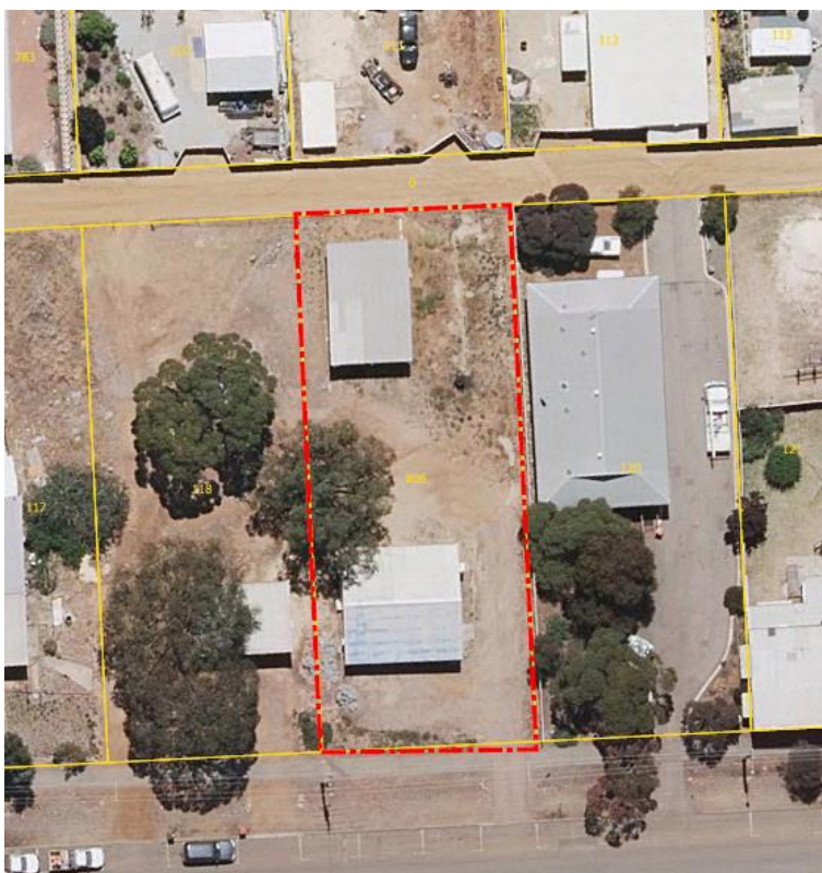
Lot 806 Morgans Street, shed at rear of the property is the subject of this application
