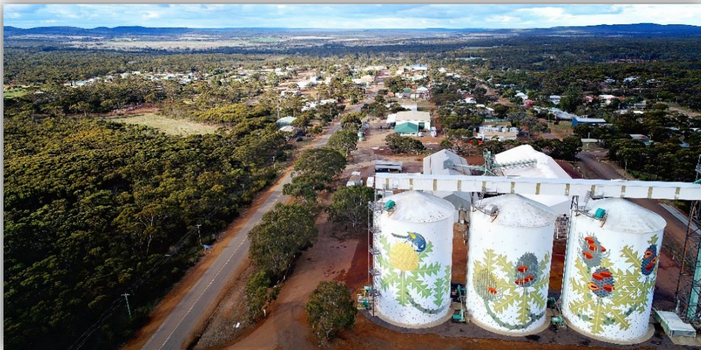
RAVENSTHORPE TOWNSITE - SILOS
