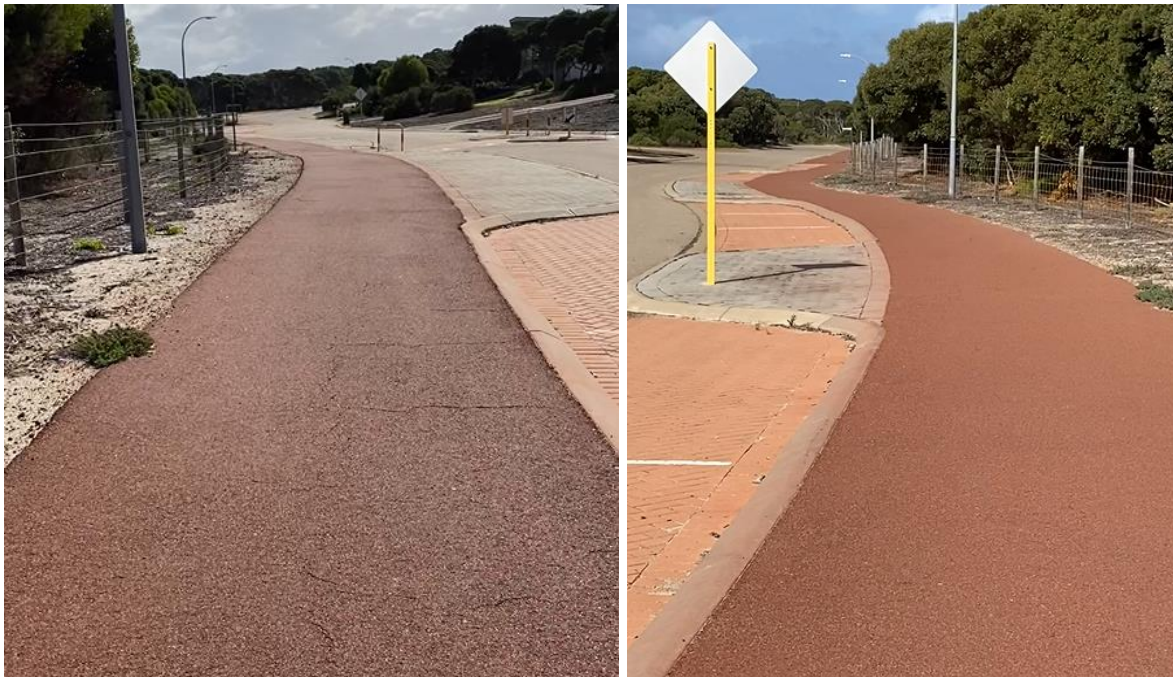
Figure 4-50: Canning Boulevard from Kepler Street
