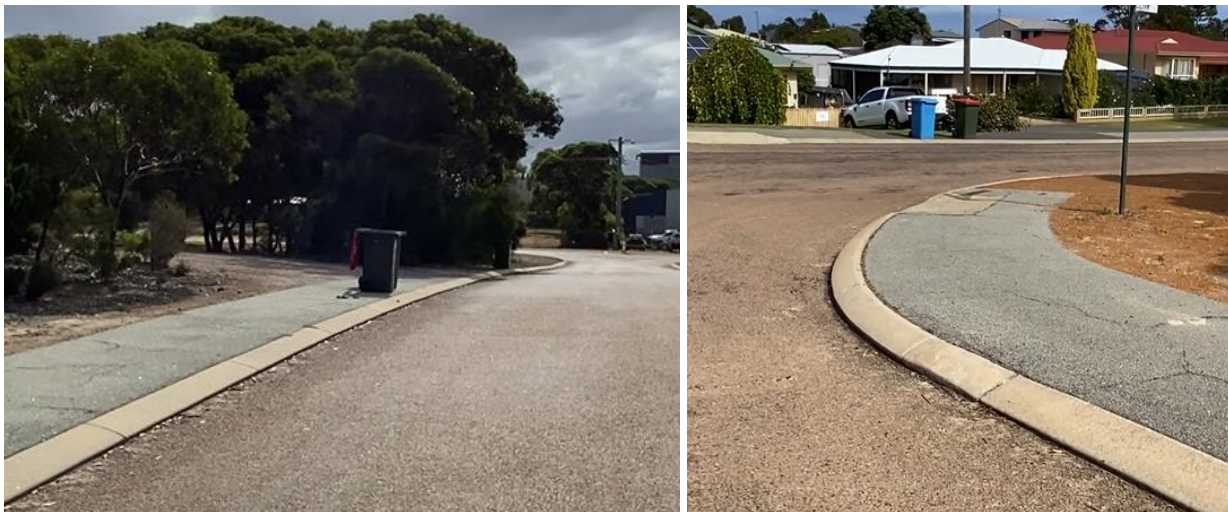
Figure 4-40: Hakea Street from Tamar Street
