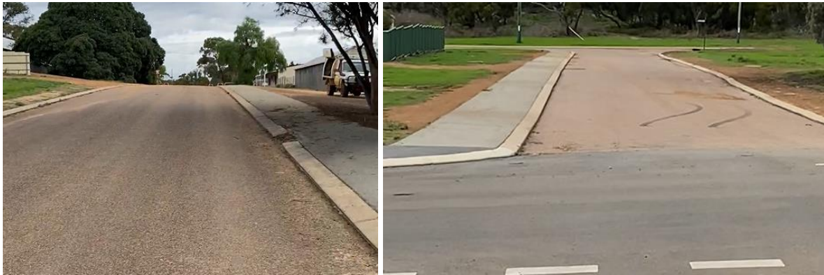
Figure 4-20: Andre Street Path Network between Morgans Street and Spence Street
