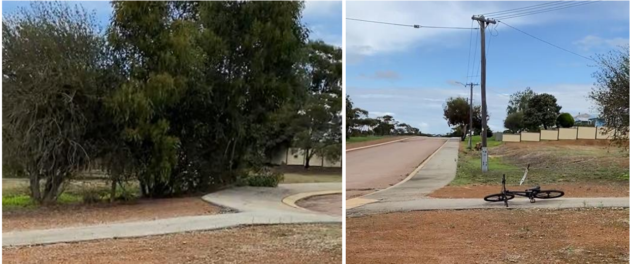
Figure 4-78: Tubada Street West at Cul de Sac
