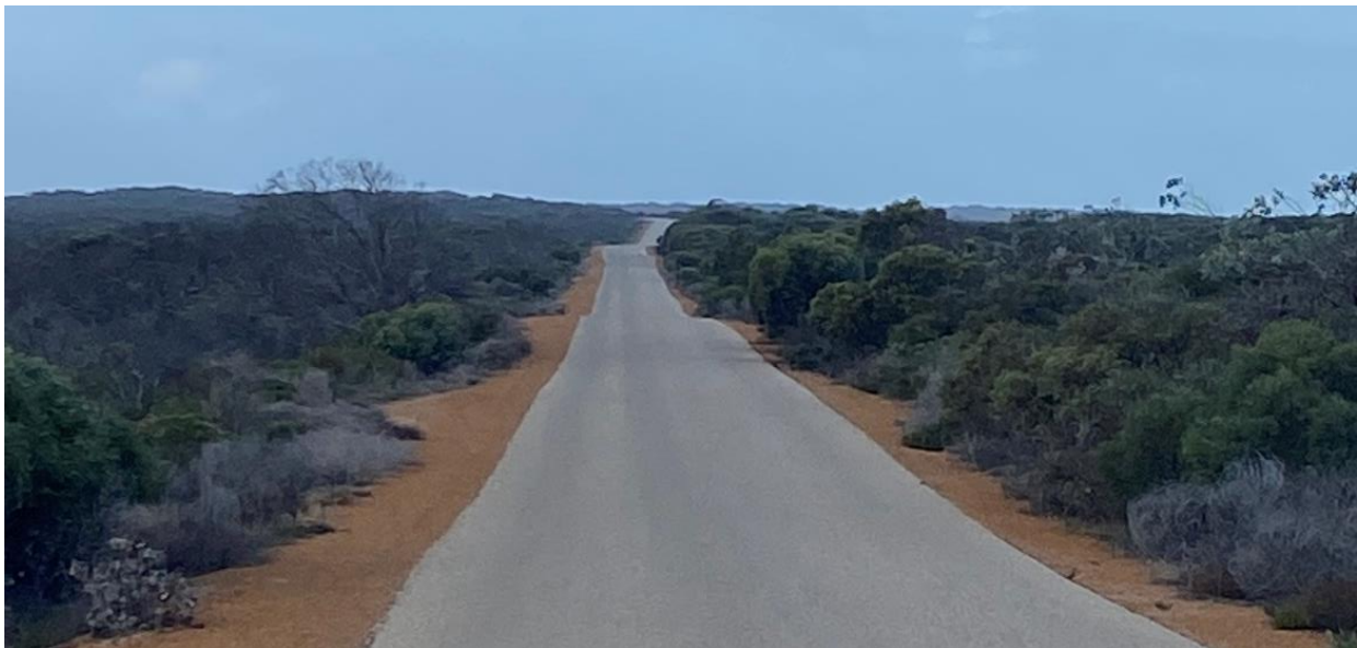
Figure 4-72: Southern Ocean Road from Esplanade East
