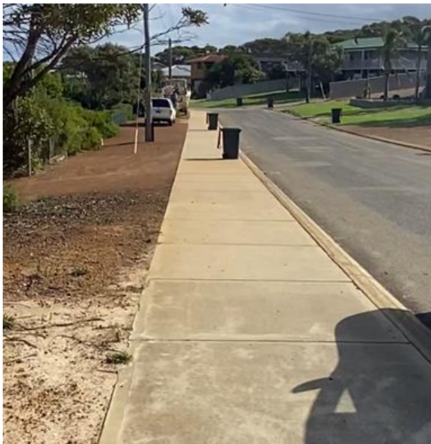
Figure 4-58: Birdwood Street from Wilkinson Street
