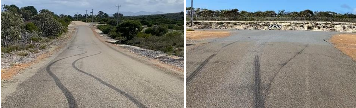
Figure 4-35: Banksia Road from East of Boroonia Street
