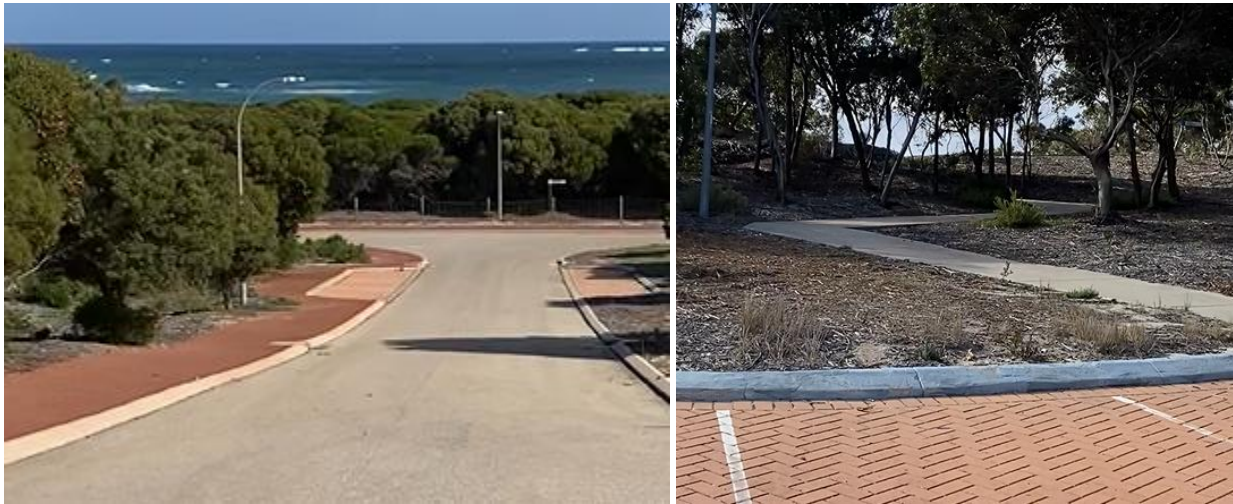
Figure 4-55: Marloo Grove from Barrens Way
