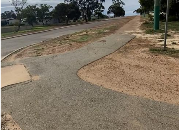
Figure 4-29: Daw Street from Carlisle Street
