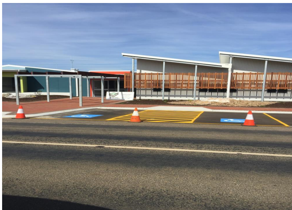
Photo: New Hopetoun Community Centre Disabled Parking Bays and Access Ramp
