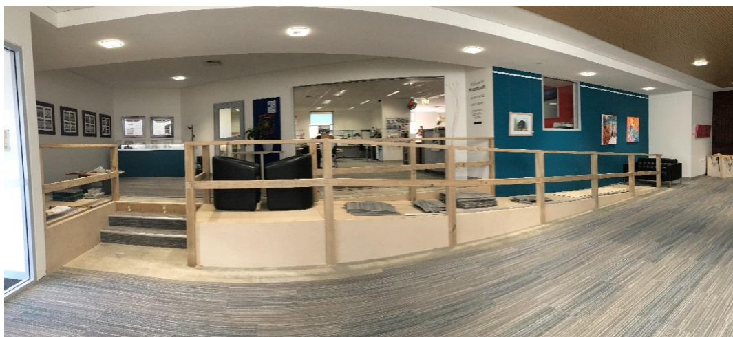
New ramp during construction
