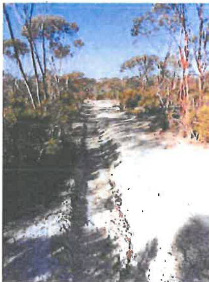
Erosion on the trail surface leading into Kundip townsite from the west
